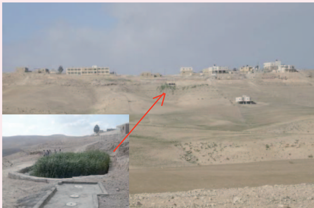
Figure 2: Greywater treatment CW in Al-najada, Hebron district, Palestine.
