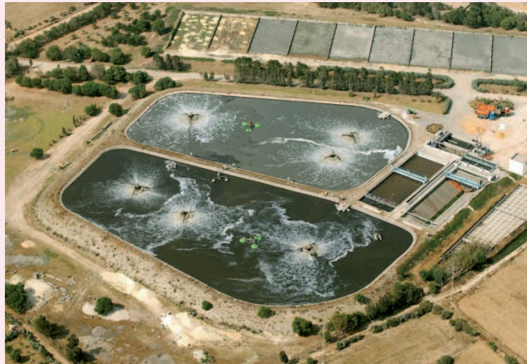
Figure 4. The Mahdia WWTW (aerated pond system), in Tunisia. It is designed for 150,000 population equivalent (Real flow rate: 426 m 3 /h). Treated water is UV-disinfected before discharge (Al Ayni, 2012).
