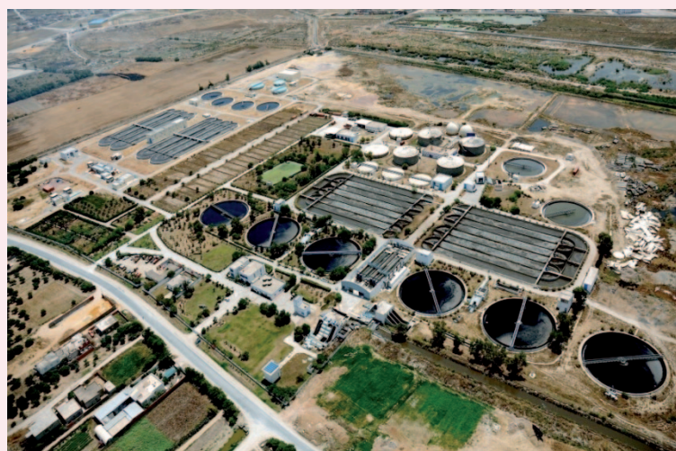
Figure 2. The Choutrana wastewater treatment complex (activated sludge + anaerobic digestion of excess sludge) in Tunisia. The 2 WWTPs, designed for a total of 1,300,000 population equivalent. Real flow rates: 3,250 m 3 /h for the oldest, 1,667 m 3 /h for the most recent (Al Ayni, 2012)
