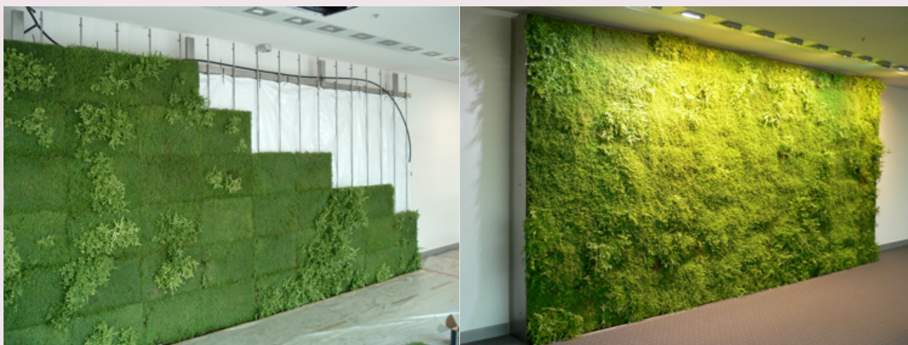
Figure 2. Green Wall Sparkassa Ingolstadt: modular system (left) and later the connate plates (right) (photo by B. Häring)
