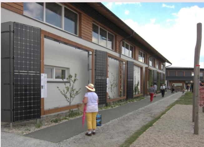
**Figure 2.** The GruenAktivHaus-lighthouse project at Sonnenwelt, Grossschoenau, Lower Austria, Austria. Participants of the new developed training course used their new learned knowledge to plan and construct this building project presenting innovating synergies and usage of living walls and green roofs, solar energy technology, LED technology and solar architecture.
