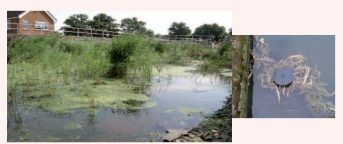
Figure 1: Example of subsurface flow wetlands with surface flow during high flow conditions. The water flows preferentially over the top of the bed and will result in partially treated water exiting through the overflow pipe and blending with the treated effluent at the final collection point.
