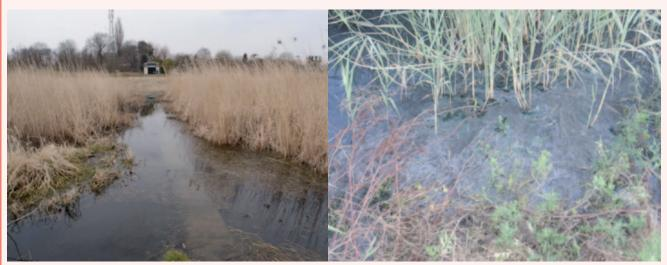
Figure 4: Examples of clogged horizontal flow wetlands (a) Hydraulically linked UK tertiary wetland cells and (b) Surface ponding and hydrogen sulfide generation in secondary wetland in Italy. Picture (b) courtesy of IRIDRA Srl.
