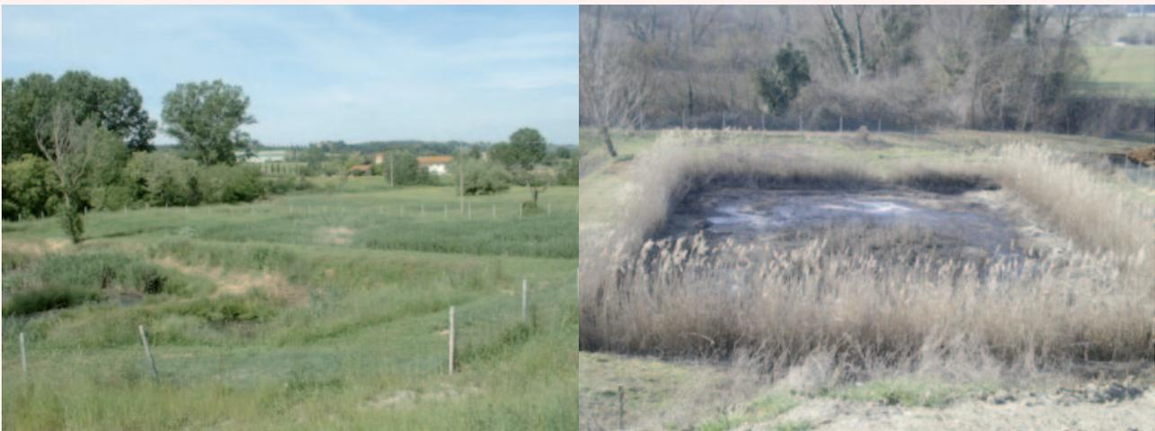
**Figure 6: Winery horizontal flow wetland (a) before and (b) after clogging developed. The loading rate onto the wetlands was three times the design load by the time clogging became permanent. Images courtesy of IRIDRA Srl.**
