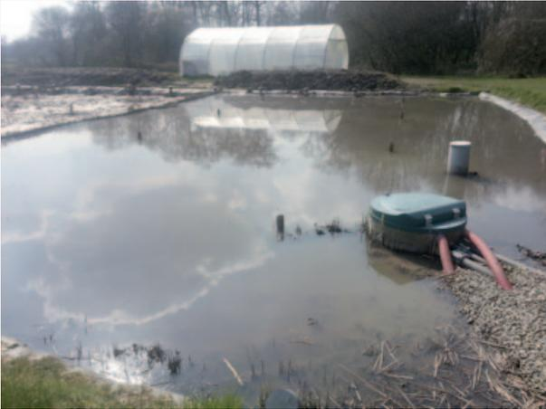
**Figure 7: Example of 1<sup>st</sup> stage clogging in a VF CWs system.**
