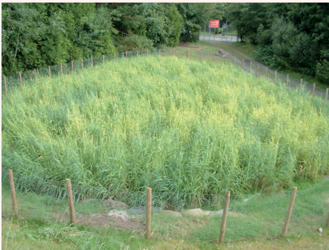
Figure 3a: Pont Abraham reed bed, during first growing season, receiving well aerated RBC effluent (diluted with groundwater infiltration), showing yellow reeds throughout (13Aug08)
