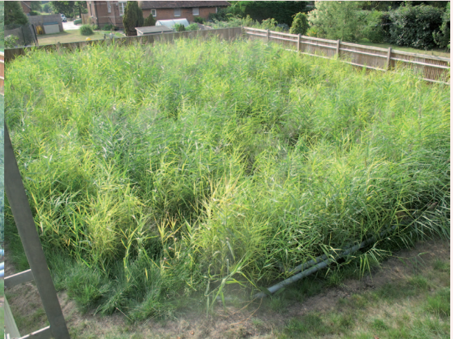
Figure 2b: Bodiam Castle reed bed, third season, with effluent recirculation, showing less dense, yellow reeds throughout (even following ferrous sulphate foliar spray on 16Jul13) (22Aug13)
