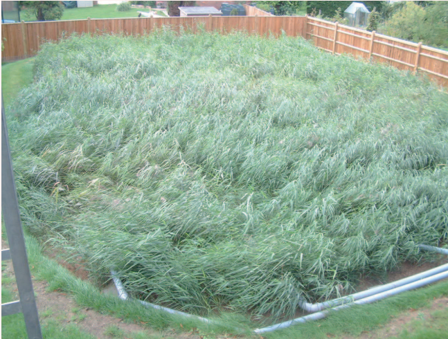
Figure 2a: Bodiam Castle reed bed, during first growing season, with no effluent recirculation, showing dense, green reeds throughout (12Sep11)
