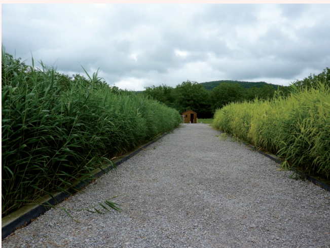
Figure 4a: Floirac first and second stage French system reed bed (left & right, respectively), showing yellowing of leaves in second stage, compared to vigorous green leaves in first stage (courtesy Joëlle Paing)
