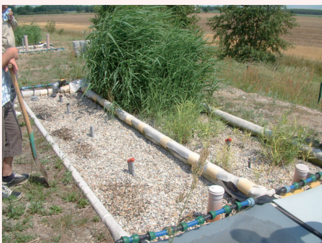
Figure 5a: Langenreichenbach horizontal flow forced aeration reed bed, receiving settled effluent: tall, green, dense reeds near inlet; short, yellow reeds further from inlet (1Jul11)
