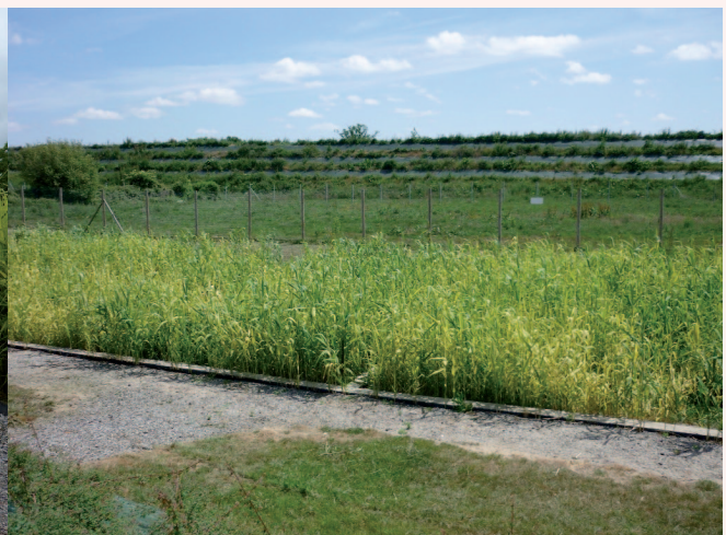
Figure 4b: Hauterive second stage French system reed bed, May 2011, receiving vertical down-flow reed bed effluent treating raw sewage, showing some yellowing throughout bed (courtesy Joëlle Paing)
