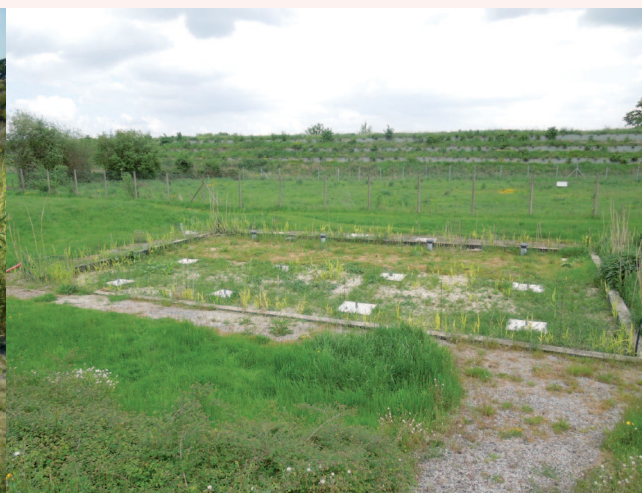
Figure 4d: Hauterive second stage French system reed bed, May 2013, almost complete disappearance of reeds within three years of first yellowing, with replacement by “weeds” (courtesy Joëlle Paing)
