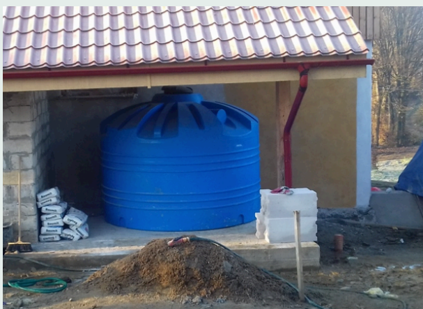
Figure 6. Rainwater harvesting system in Nijne Selishe during construction. (source: ESF)
