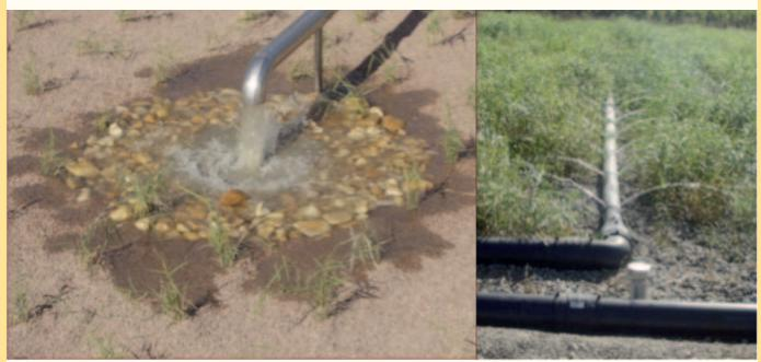
Figure 6: First stage feeding device (Epur Nature)
