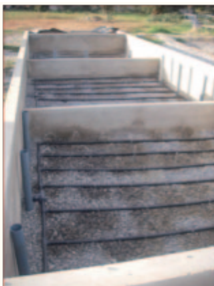
Figure 7. Tertiary VF Sand Filter Cross Photo (2011)
