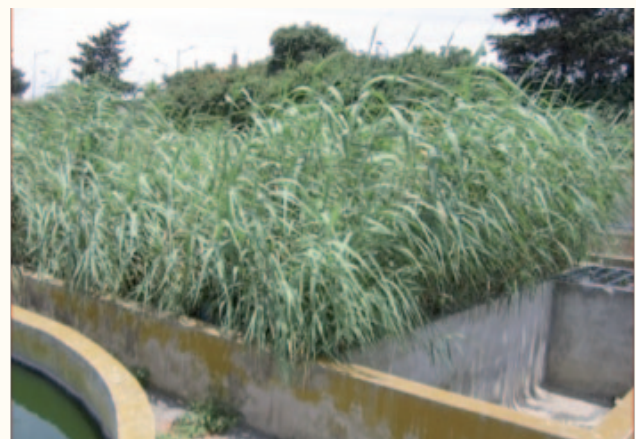
Figure 3: Primary VF Wetland - Photos (2007, left, and 2011, right)
