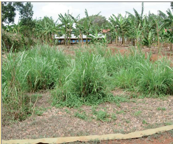
**Picture 4: Horizontal flow CW system in Kalungu.**
