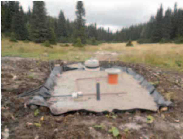
Figure 5: Vertical flow constructed wetland (left) and the layers of the vertical flow bed (right).
