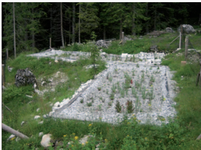
Figure 8: The constructed wetland system (Picture: G. Langergraber).
