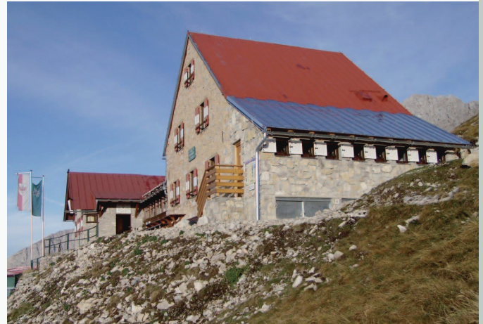
Figure 3: Bettelwurf Hütte with new sanitation facility and chambers for faecal matter (lower right corner) (Picture: Amor, 2006).
