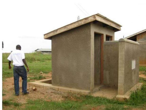
**Figure 5: UDDT toilet with underground faecal chambers in Kitgum.**
