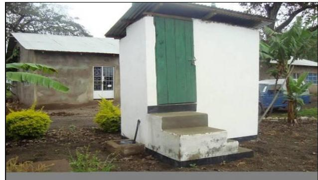
**Figure 1: Front view of the Nanenane UDDT: 20 litres urine tank adjacent to the door.**
