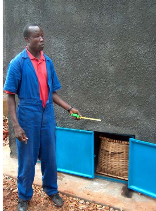
Picture 6: dry toilets; backside with door and basket for faeces
