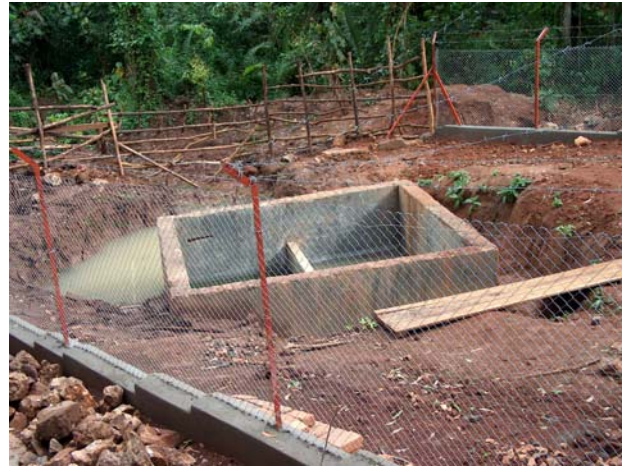
Picture 12: catchment chamber during construction
