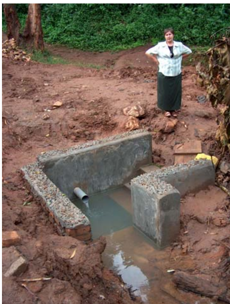
Picture 13: Spring overflow during construction
