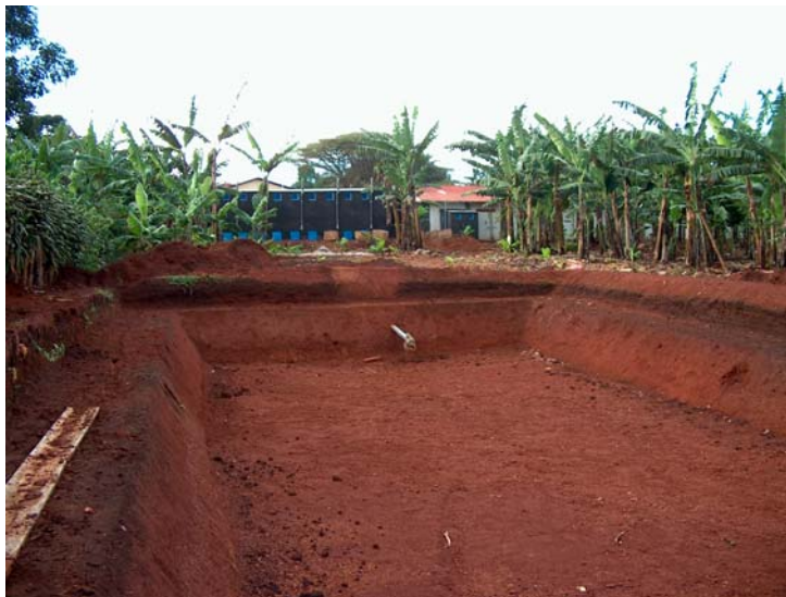
Picture 8: Constructed wetland system during construction
