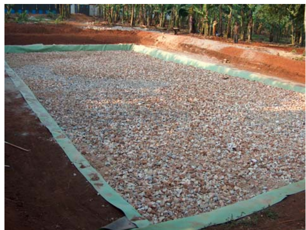
Picture 9: Constructed wetland completed (not yet planted)
