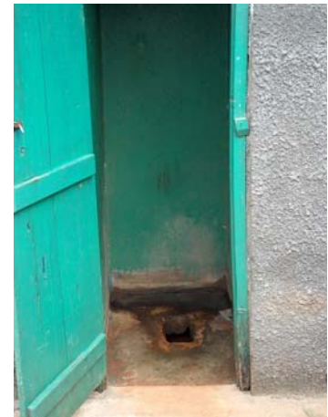
Picture 2: old pit latrines
