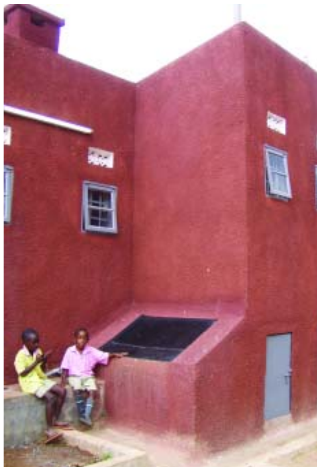
A dry toilet constructed inside a house (St. Franzis Naggalama Hospital/Uganda)
