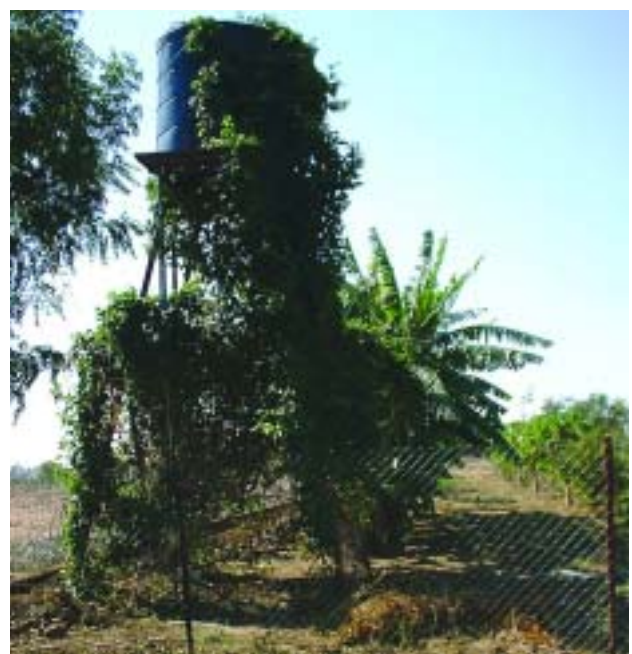
Tank with treated wastewater for irrigation (Matany Hospital/ Uganda)
